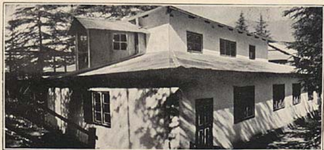
A VIEW OF THE NEW BUILDING FROM THE N.E., SHOWING BRIDGE LEADING TO THE ROCKS.
