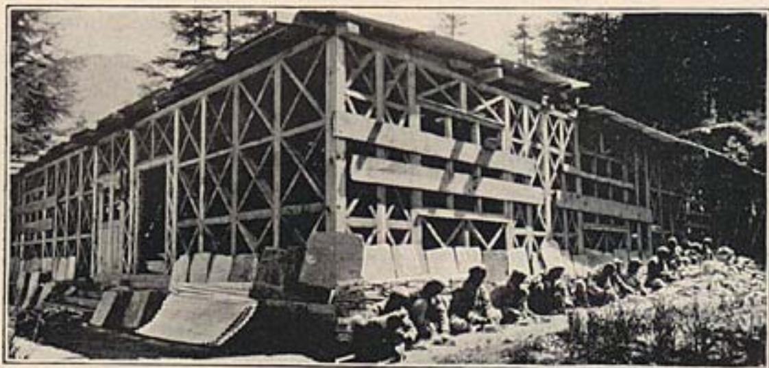
THE EARTHQUAKE PROOF DHAJJI DIWAR CONSTRUCTION.
