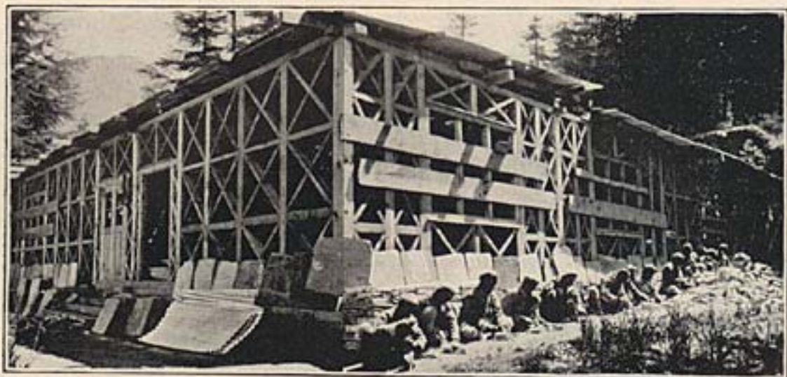
THE EARTHQUAKE PROOF DHAJJI DIWAR CONSTRUCTION.
